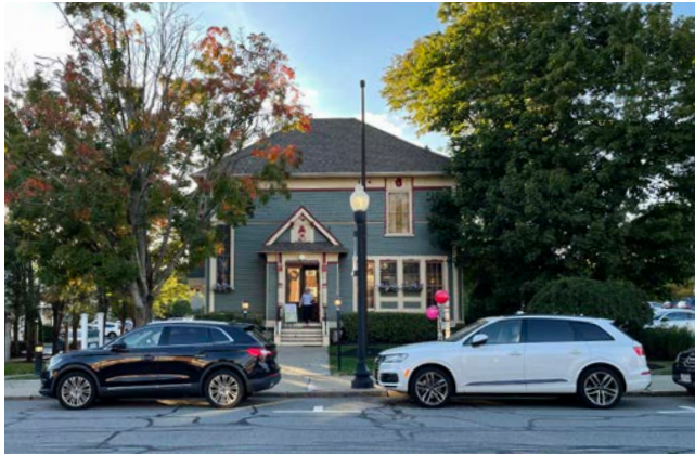
Figure 6. Current Downtown Canton character and building type examples
